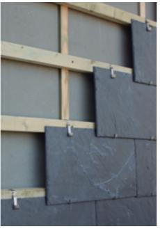
\*SLATECLAD<sup>™</sup> exclusive system uses size 60x30 CUPA natural slates laid horizontally.
